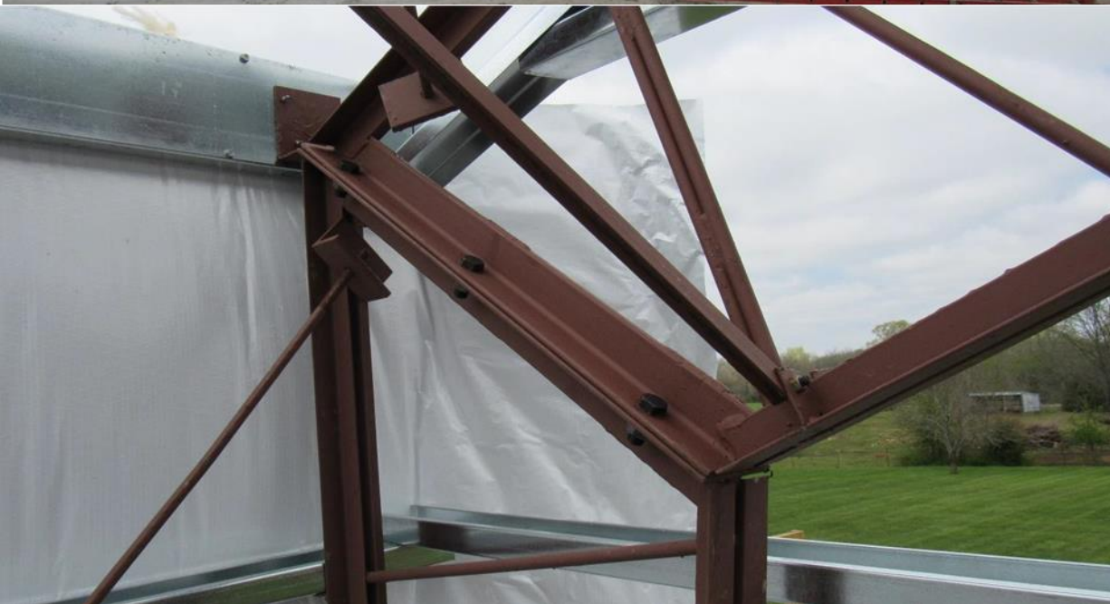
(Truss and Column at Knee Connection)
