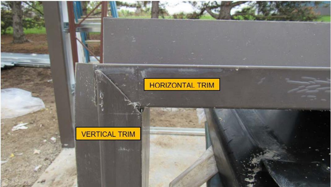
(Above is how trim will install together.)
