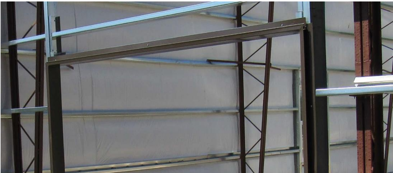
(Overhead door finished trim.)
