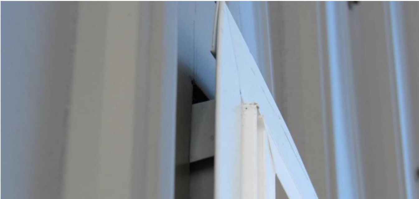
(Finished door and window trim.)
