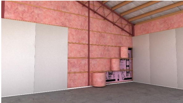
Insulate and sheet rock walls
