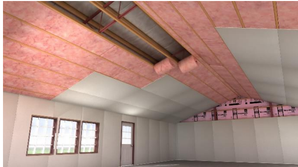
Insulate and sheet rock ceiling
